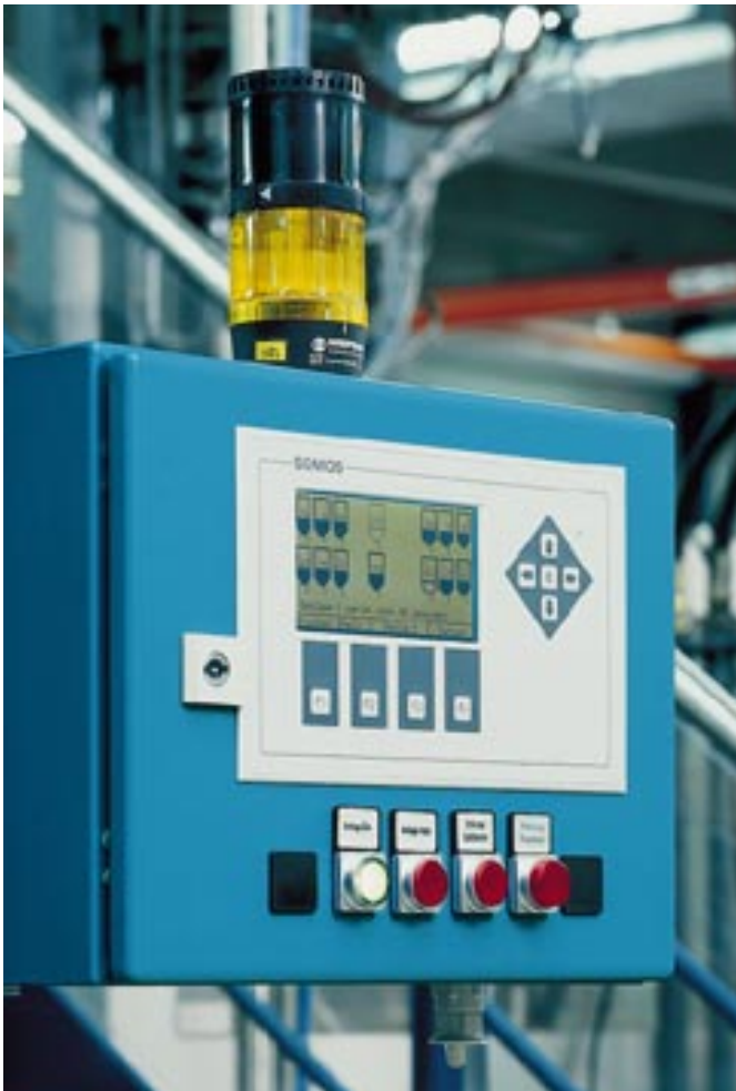
External operating panel of a control unit MC2-DIGSY
