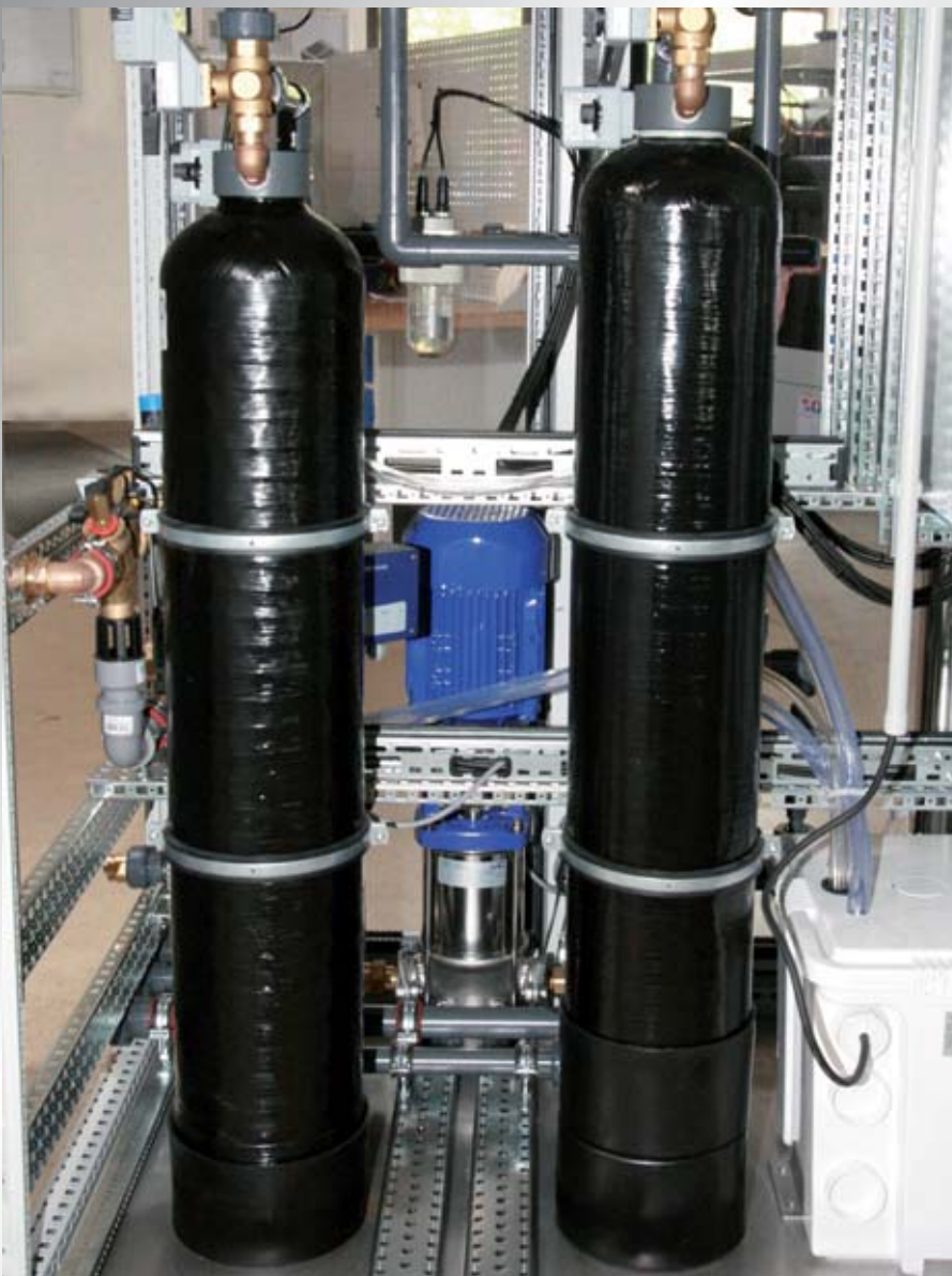
A view of the multi-stage filter unit equipped with backwash AFM and ultra-superfine filters.
