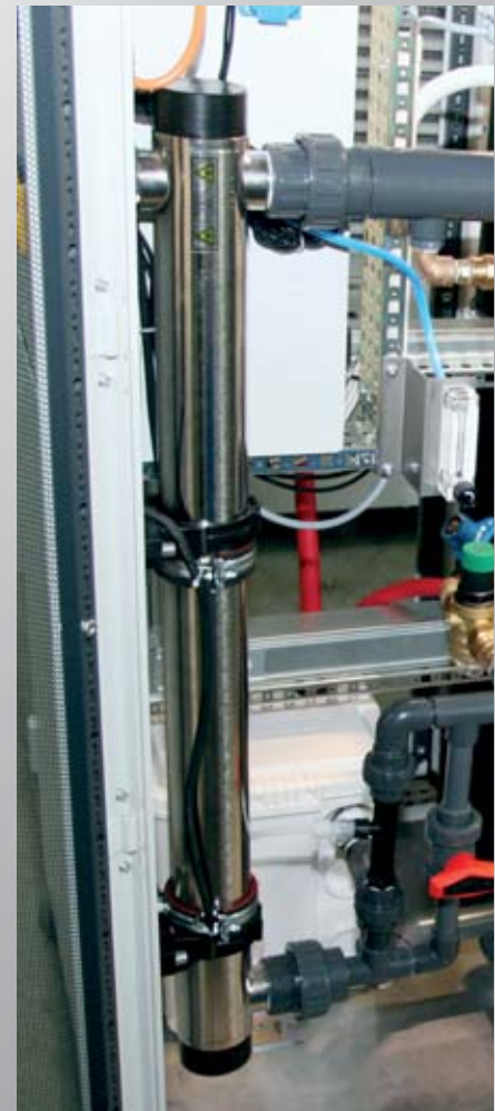
A view of the ozone reactor which is integrated into the ONI-AquaClean device and provides additional hygienic safety.
